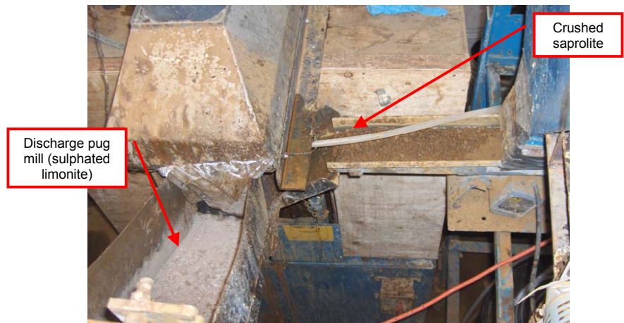
Figure 7 Photograph of Ball Mill Feed Trough
